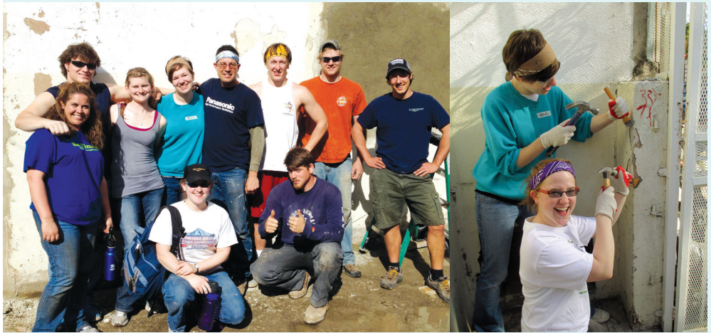
Left: Final picture of Carroll volunteers on the Habitat build site, with their building supervisor and a local AmeriCorps volunteer—the gray square in the background was a hole when the group began the week: Carroll students chipped stucco, measured and filled with plywood and three coats of stucco; Right: Mariah Ramirez, '13 (standing), and Shannon Schober, '14, carefully chip away stucco from a brick wall
