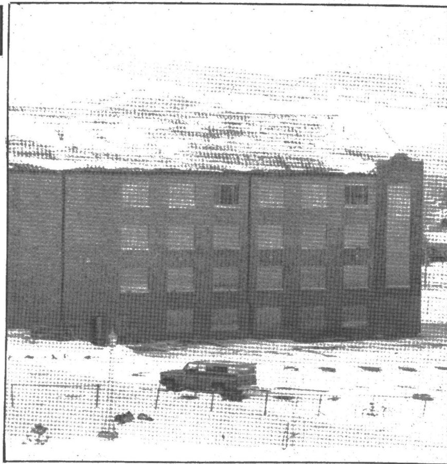
With boarded windows, Guadalupe stands empty. photo by Hisashi Tagaya
