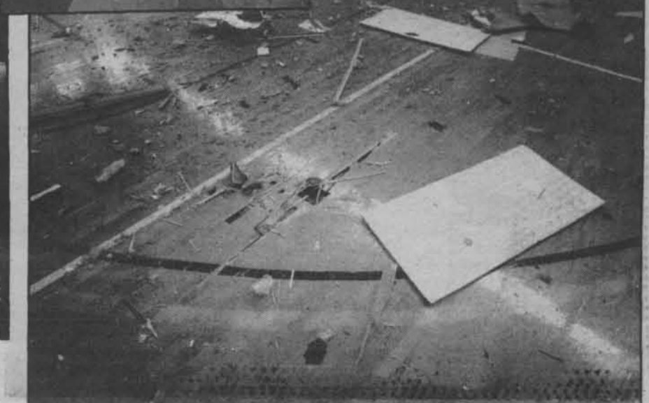
One chunk of debris gouged a hole in the floor.
