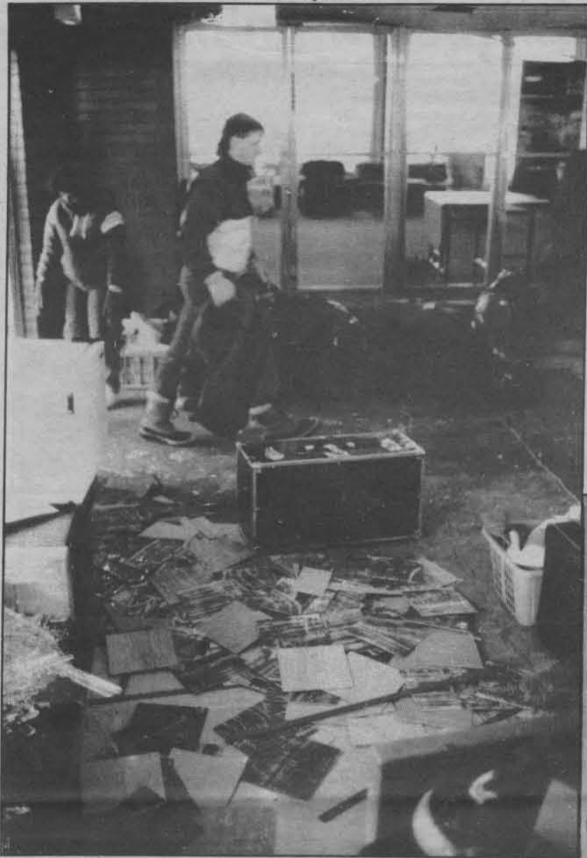
It was so cold in Guadalupe Hall, that the floor tiles began to come unglued and pop off, creating an additional mess to clean up beyond the glass which was frozen to the floor.
