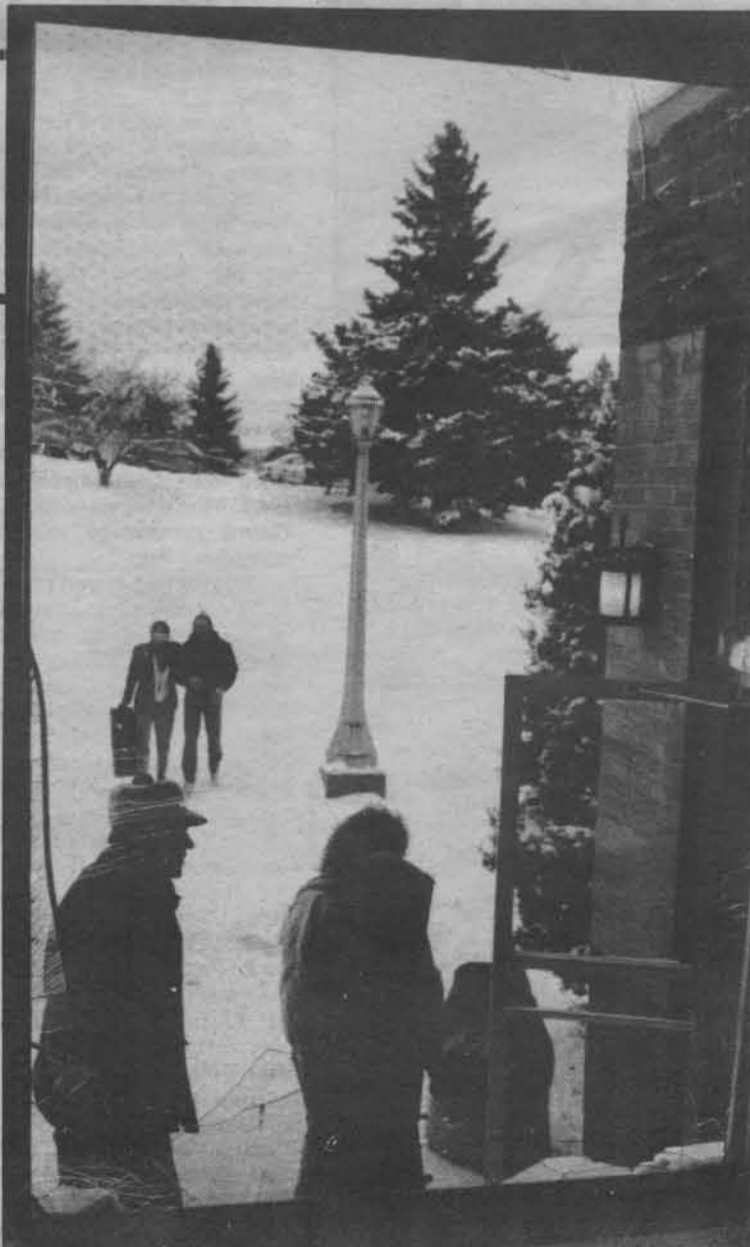
Windows on both sides of the Guad lobby had been blasted out.
